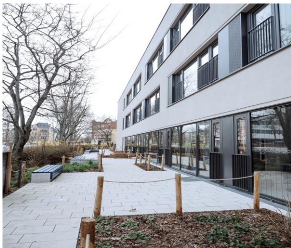
external view of the facility
